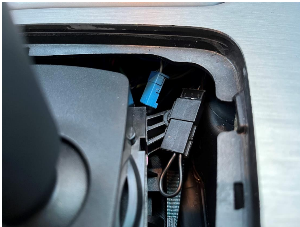
PLOCK fault rectified using a terminated loop 4-pin connector (included in the PnP harness)
